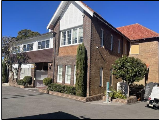
Figure 10. External view to the Jubilee Building, facing south towards the primary façade.
