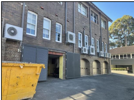
Figure 12. External view to the Jubilee Building, facing north towards the rear façade.
