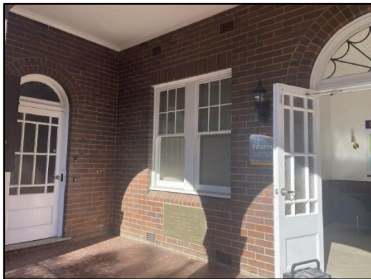
Figure 18. External view to the front verandah of the Woolwich Building.
