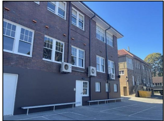
Figure 17. External view to the Woolwich Building, facing north towards the rear façade.
