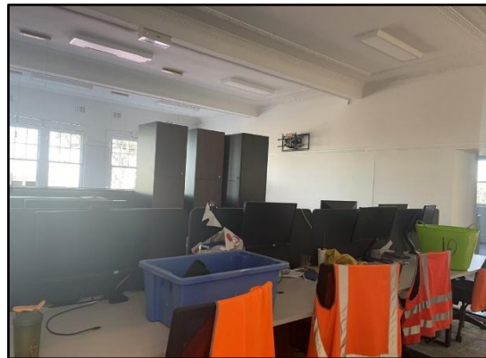
Figure 19. Internal view to the open admin area, on the Ground Floor.
