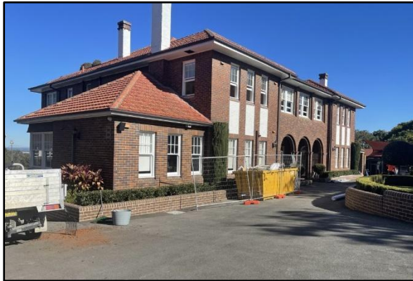
Figure 16. External view to the Woolwich Building, facing south-west.
