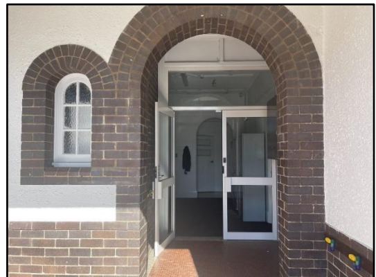
Figure 13. External view towards the front entrance to the Jubilee Building.
