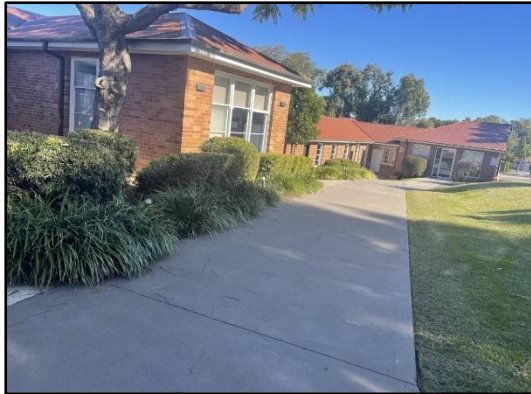
Figure 22. External view to the auxiliary buildings, facing west featuring the c.1955-1965 built forms.
